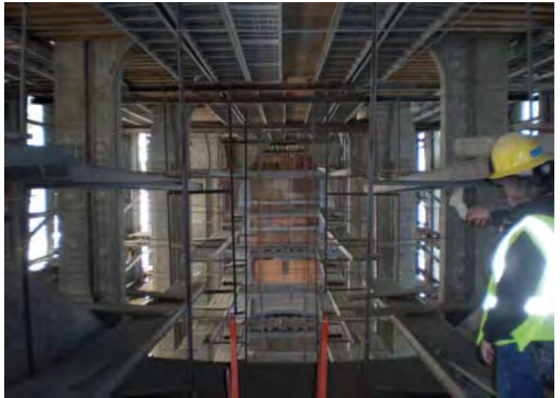
Inside the enclosure, showing the various levels and work platforms
