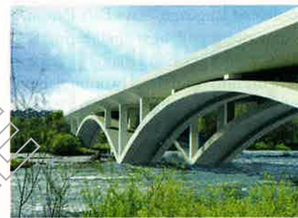
ARCHED CROSSING New Willamette bridge piers will touch down in the river at only one point.
