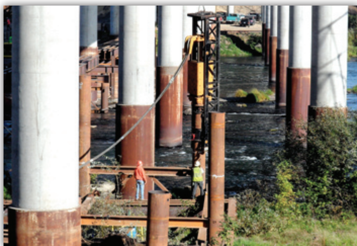
Hydraulic mechanisms at WRB use canola oil instead of petroleum-based products to reduce risk to the environment. The amount of oil it takes to cook your Holiday turkey will keep this impact hammer going for about six months. (from left) Veril Humbert and Mike Sheeley running the Hydraulic Impact Hammer while building work bridge.
